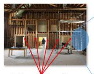
5 of 8 posts that will extend from foundation to the roof as part of the seismic upgrade.
