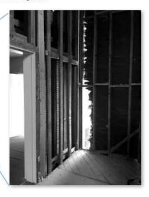
From this corner the plywood seismic "girdle" will extend to connect this part of the building with the wall from which the stucco has been removed.
